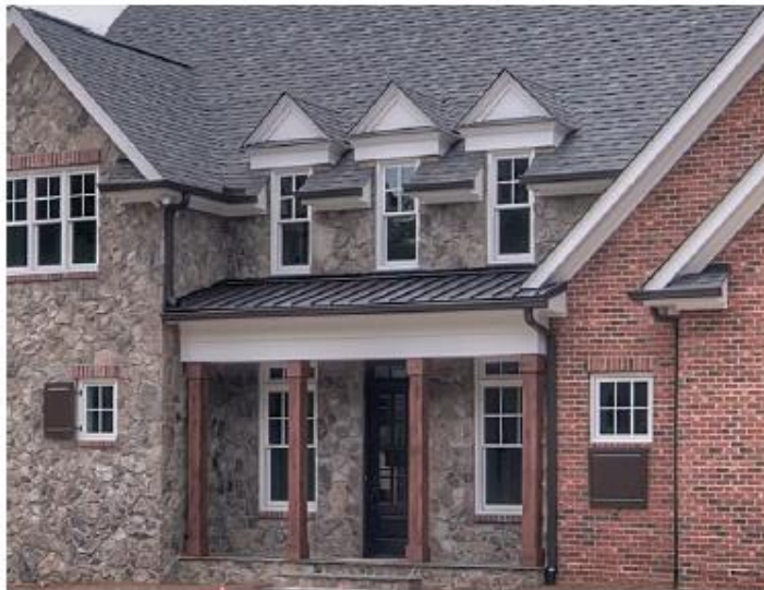
Standing Seam Metal Roofing ~ Dark Bronze
