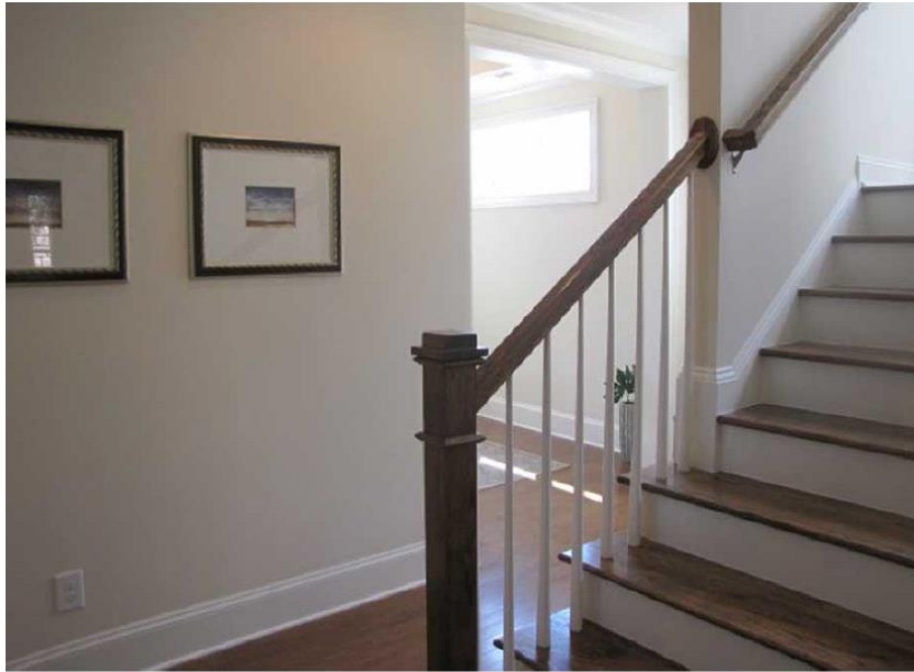
Paint Grade Balusters, Stain Grade Oak Newels with Stain Grade Oak Handrail
